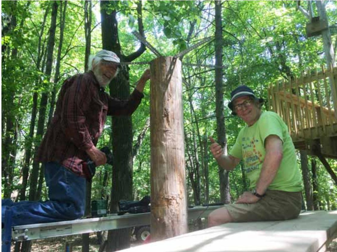
Alan and Rick are arranging long steel strips on the pole in the correct places for making a hexagonal shaped deck, and that allowed Rick and Jerry to fasten a 2 X 8 stringer to each strip so they hung off the pole in the proper places. The camp provided scaffolding and platforms for us to sit and stand on as we worked overhead.
